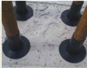
**Protects the bolt from contact with grout and prevents grout from going down into the bolt sleeve.**
